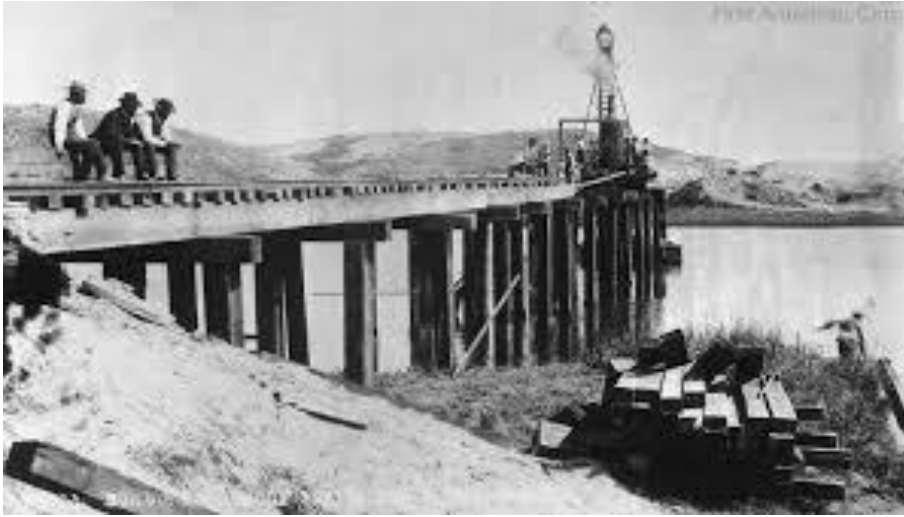
Santa Ana & Newport RR under construction.
