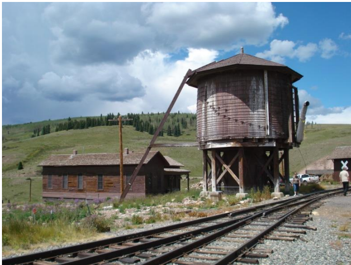
Bunkhouse and water tower at Osier
